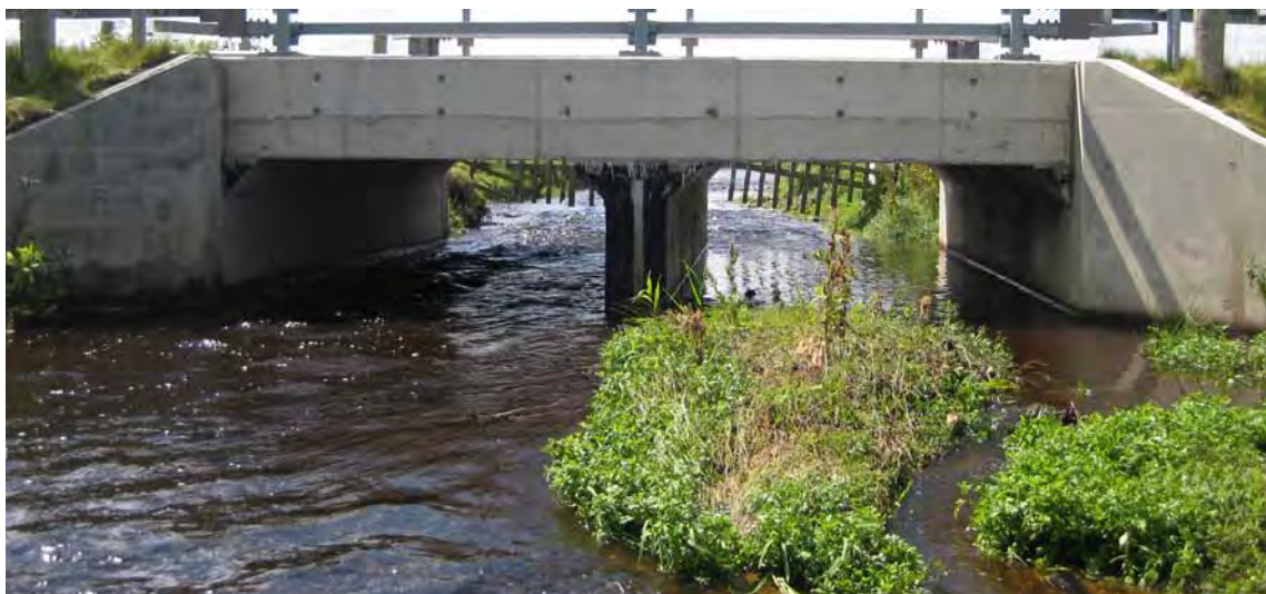
Figure 43: Twin barrel culvert that maintains natural channel width and invert buried below the natural bed level. Should only be used where single span structure or single barrel culvert is not possible.
