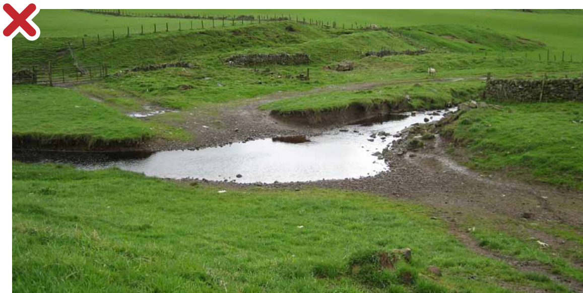
Figure 48: Poor practice, ford crossing has led to bank erosion and over-widened river. This leads to fine sediment pollution and lower water depths which are too shallow for fish to swim through, creating a barrier to fish passage.
