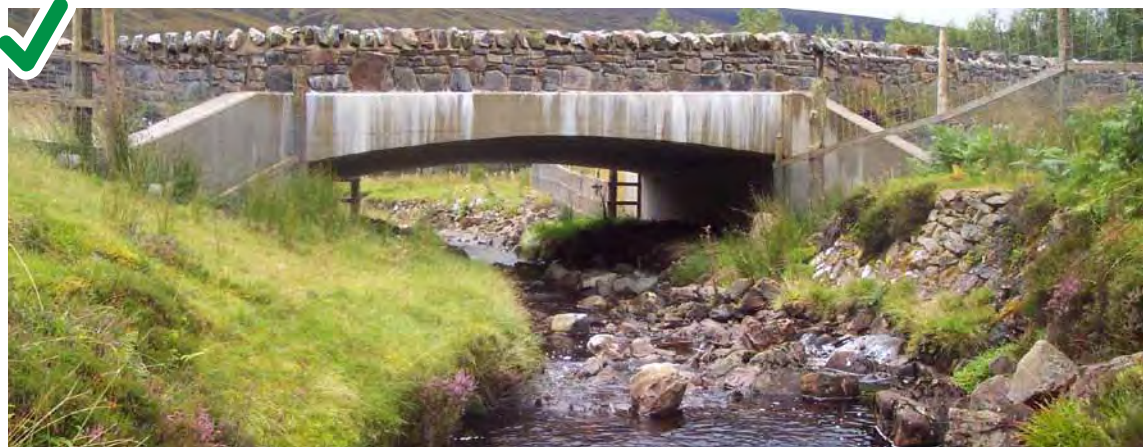
Figure 33: Good practice, bridge with piers showing set back abutments and deep foundations.
