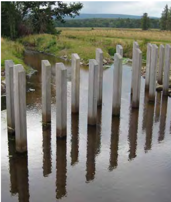
Figure 47: Trash screen bar spacing should be as large as possible (see photo on left). Smaller bar spacing can create a barrier to fish passage (see photo on right).
